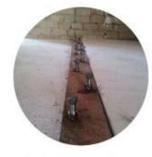
It is composed by high-strength steel, greater than 800 MPa, suitably worked with self-tapping thread in its slower part in order to improve the mechanical anchoring in the metal. It has a shaped profile in its top for joining the concrete slab.
